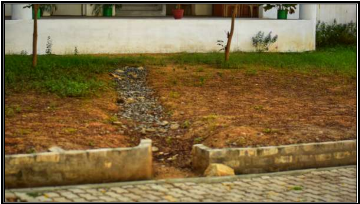
Rain Water Harvesting Pit
