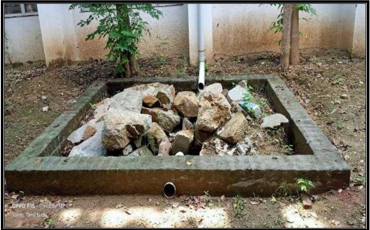
Rain Water Harvesting Pit
