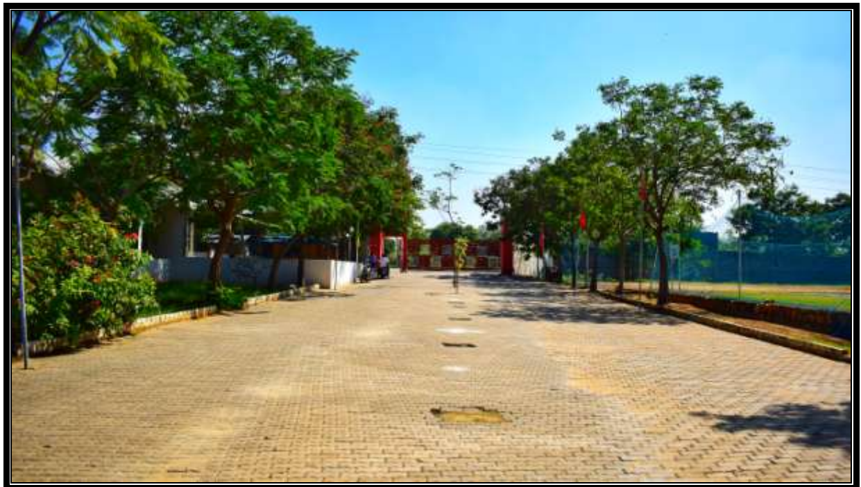
Road Having Gradient to Collect Surface Water
