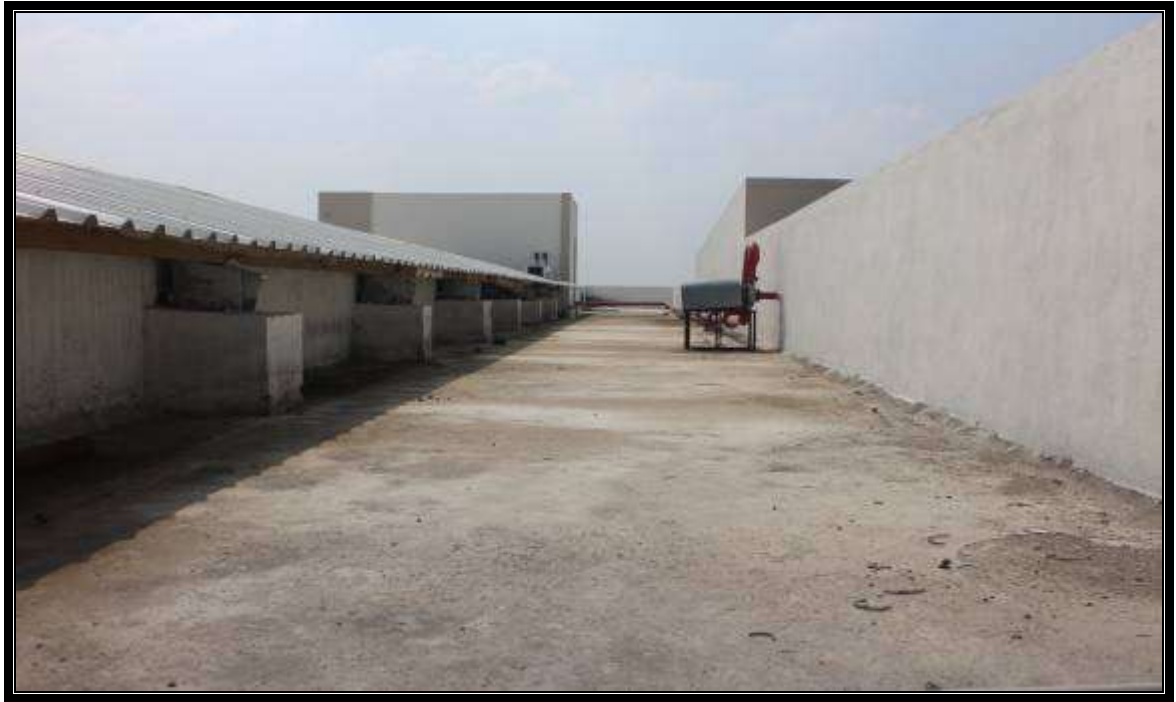
Open Terrace Finishing to Flow Rain Water to Down Take Pipe
