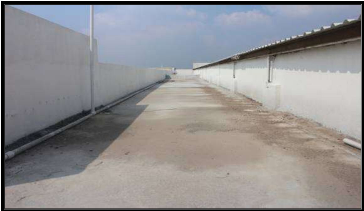
Open Terrace Finishing to Flow Rain Water to Down Take Pipe
