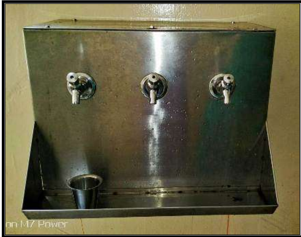
RO drinking water distribution taps
