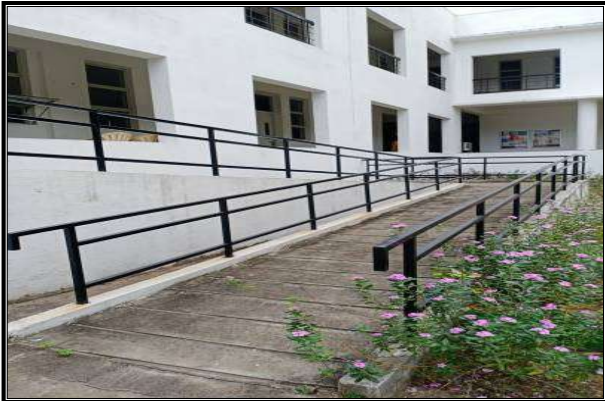
Ramp facility at DGCT new admin block
