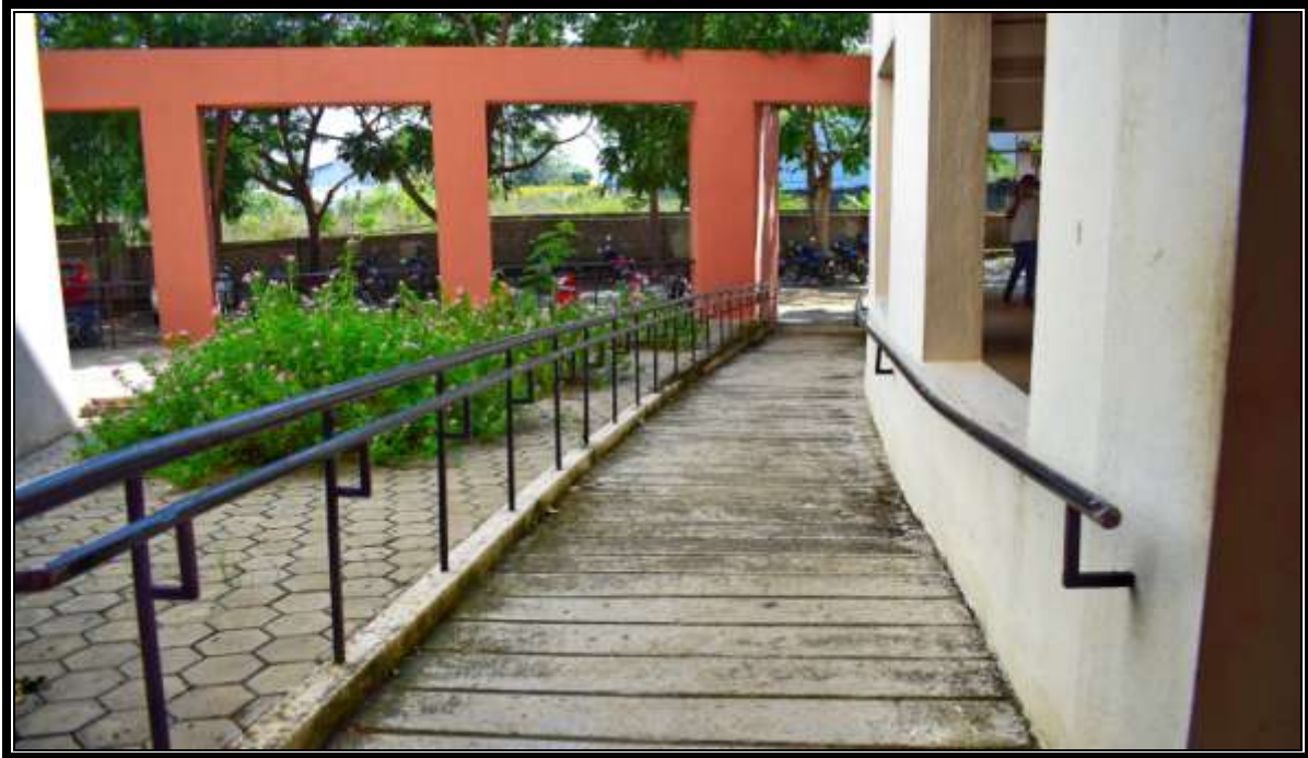
Ramp facility at DGCT main building
