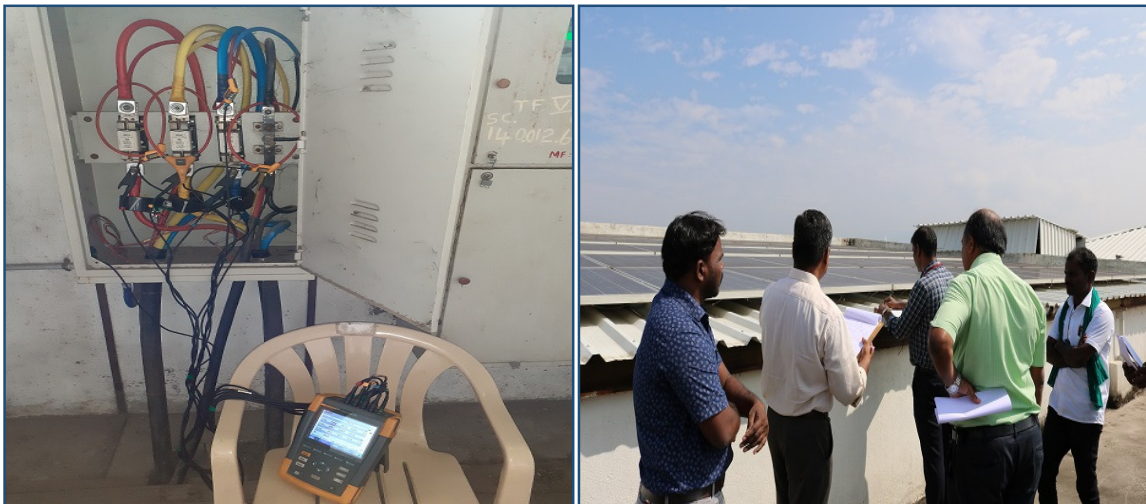
Fig. A-3: Assessment on Power House & Rooftop Solar PV System
