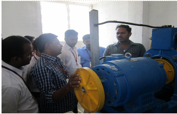
Faculty members interacted with the Service Engineer of TAMIL ELEVATORS during the Awareness Programme on 29.12.2015.
